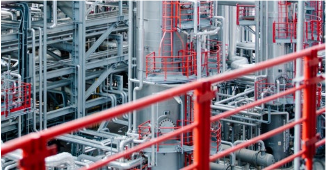
FCC modernization project
