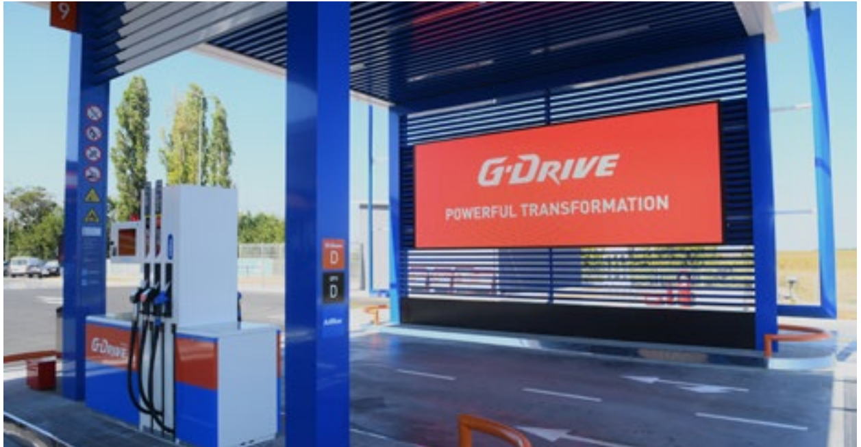
GAZPROM brand petrol station modernization
